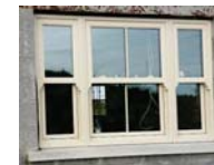
Windows - upvc cream mock sash
